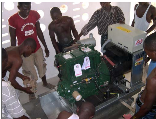
The new generator is installed at the Makeni Prosthetics Center
